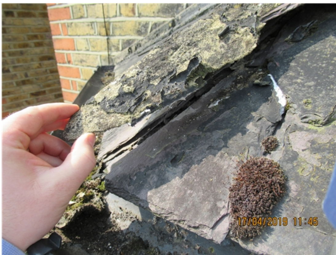
Lifting of mortar to front bay roof. Delamination to slate covering.
